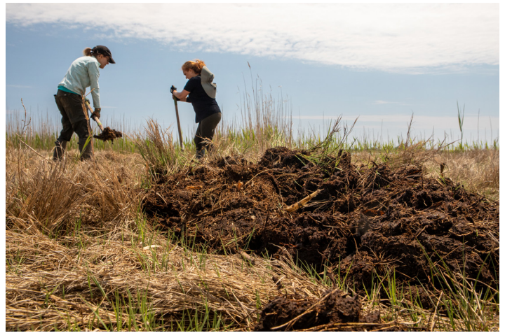
Restoration practitioners work to repair the hydrology of the marsh platform. Lauren Owens Lambert.
