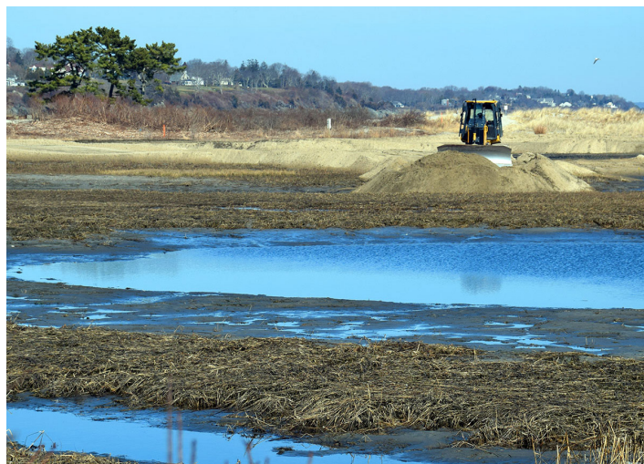
Sediment deposition on the marsh platform can help coastal marshes keep up with sea level rise. USFWS
