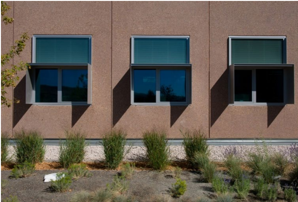
Shading was applied around the windows on the exterior of the Research Support Facility (RSF) at the National Renewable Energy Laboratory (NREL). Photo by Dennis Schroeder, NREL 19798.
