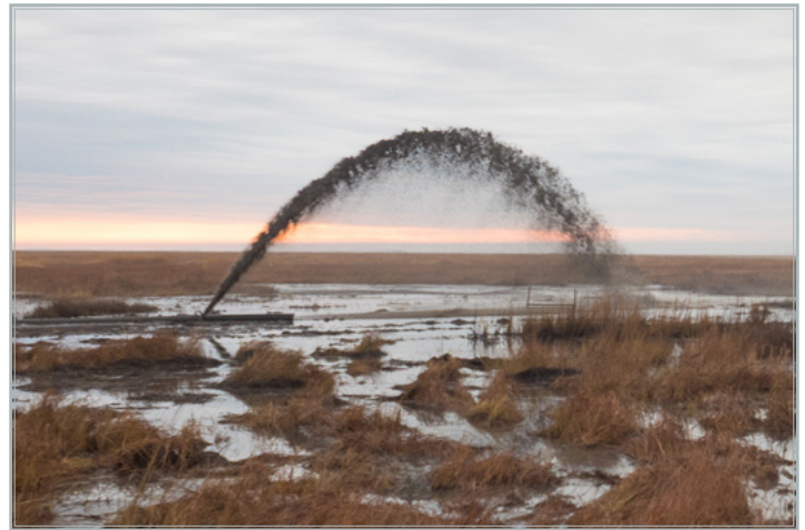
Sediment placement on the marsh platform reinvigorates the accretion process, helping marshes make up for reduced sediment input over time. USFWS
