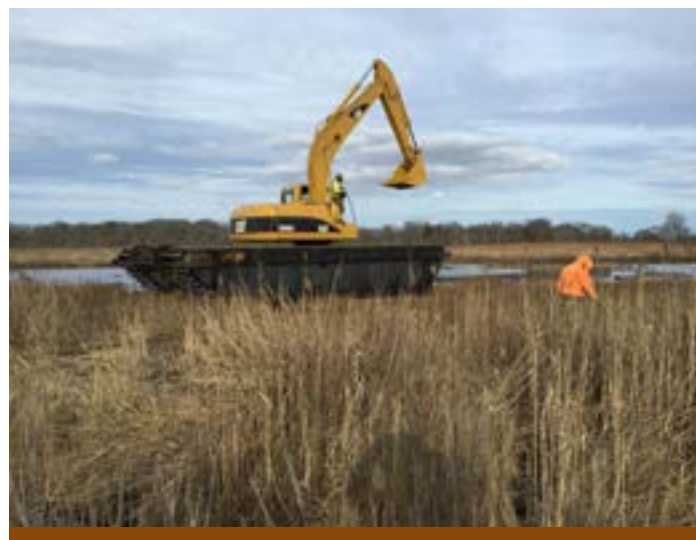
A low ground pressure excavator is moved into position on the salt marsh at Seatuck National Wildlife Refuge to spread freshly dredged sand in waterlogged section of marsh. C. Comber, USFWS
