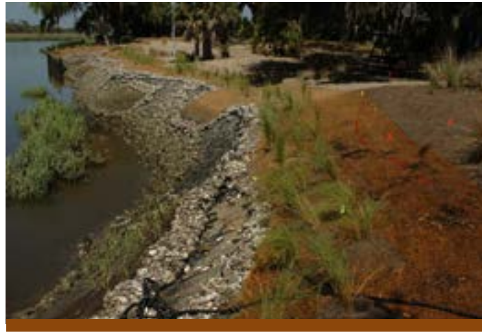
This living shoreline project constructed on Little St. Simons Island is a good example of a strategy to mitigate the effects of sea level rise and the negative effects of “hard” armoring shorelines. Todd Schneider
