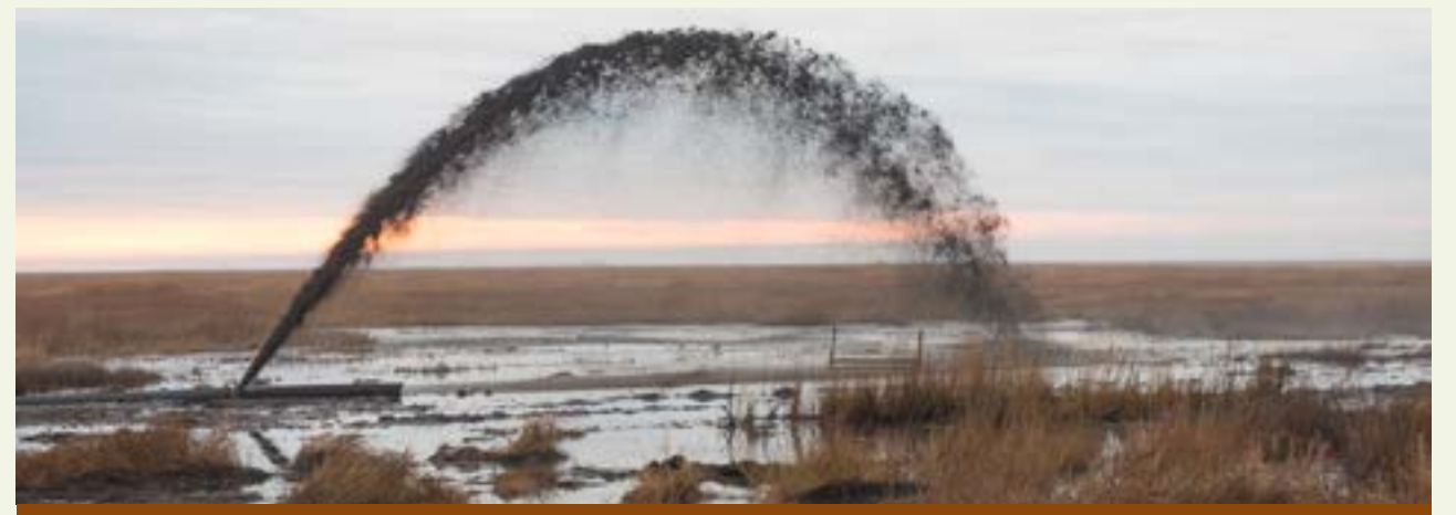
Thin layer deposition projects like this one at Blackwater NWR, spray sediments to compensate for its natural tendency to sink and the effects of sea-level rise. Dave Harp, Chesapeake Photos
