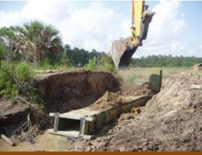
Installation of rice trunk for water level management. Joe Cockrell, USFWS
