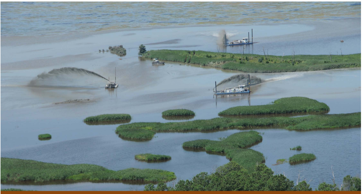
Aerial view of restoration activities at Prime Hook National Wildlife Refuge, Delaware. Richard Weiner
