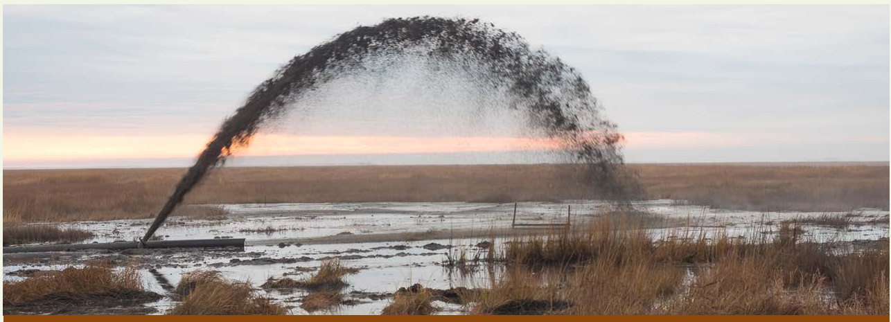
Thin layer deposition projects like this one at Blackwater NWR, spray sediments to compensate for its natural tendency to sink and the effects of sea-level rise. Dave Harp, Chesapeake Photos
