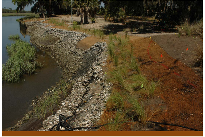
This living shoreline project constructed on Little St. Simons Island is a good example of a strategy to mitigate the effects of sea level rise and the negative effects of “hard” armoring shorelines. Todd Schneider
