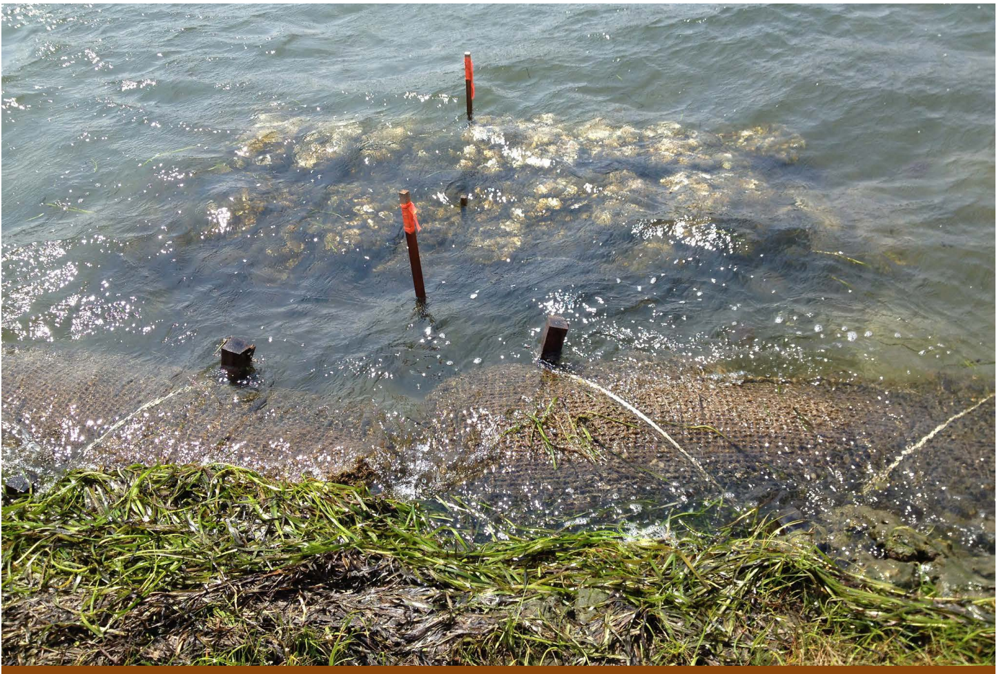
Oyster reefs, like this one built at John H. Chafee National Wildlife Refuge are an increasingly utilized technique in building living shorelines. Lia McLaughlin, USFWS
