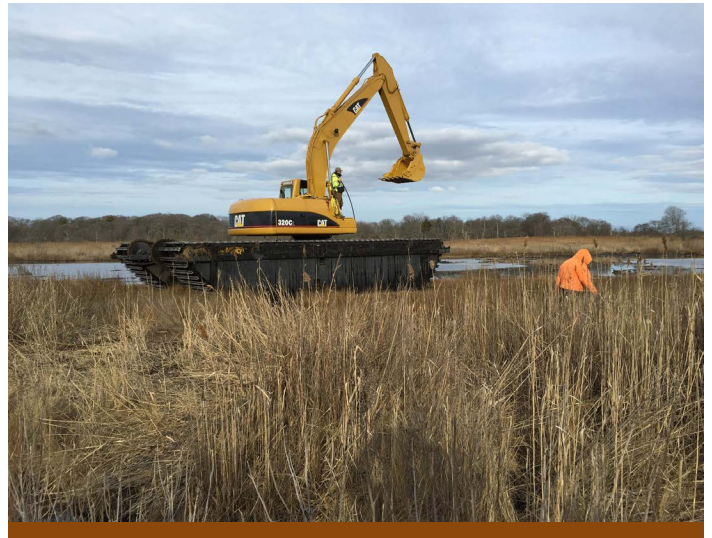
A low ground pressure excavator is moved into position on the salt marsh at Seatuck National Wildlife Refuge to spread freshly dredged sand in waterlogged section of marsh. C. Comber, USFWS
